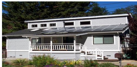
House with Solar PV System (Source: Carlsonsolar, USA)
